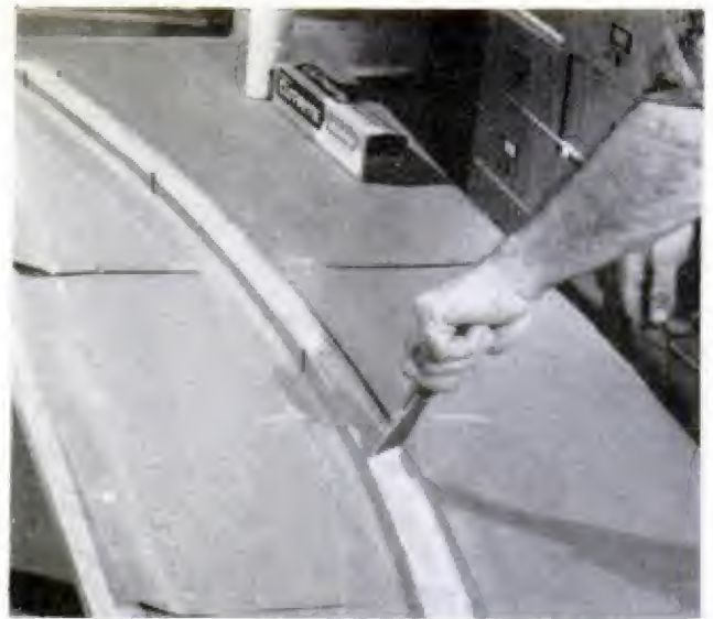
BEFORE GLUE DRIES , flex the strip to desired arch by bridging preset nails. Scrape off glue ooze-out
